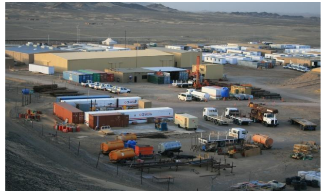
CURRENT WORKSHOP & OFFICE AREA REKO DIQ
