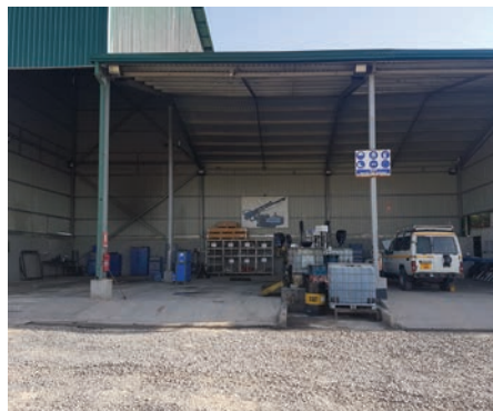
Medium term maintenance infrastructure at North Mara Gold Mine, Tanzania
