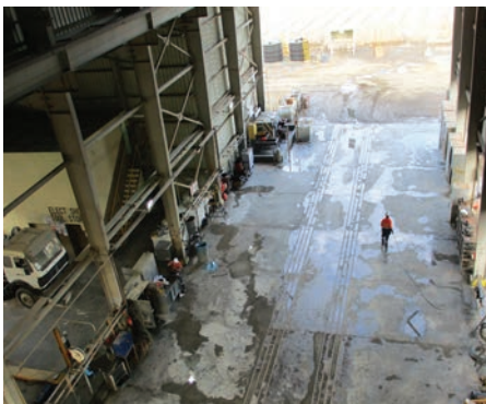
Long term maintenance infrastructure at Sukari Gold Mine, Egypt
