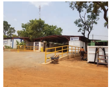
Short term maintenance infrastructure at Syama Gold Mine, Mali
